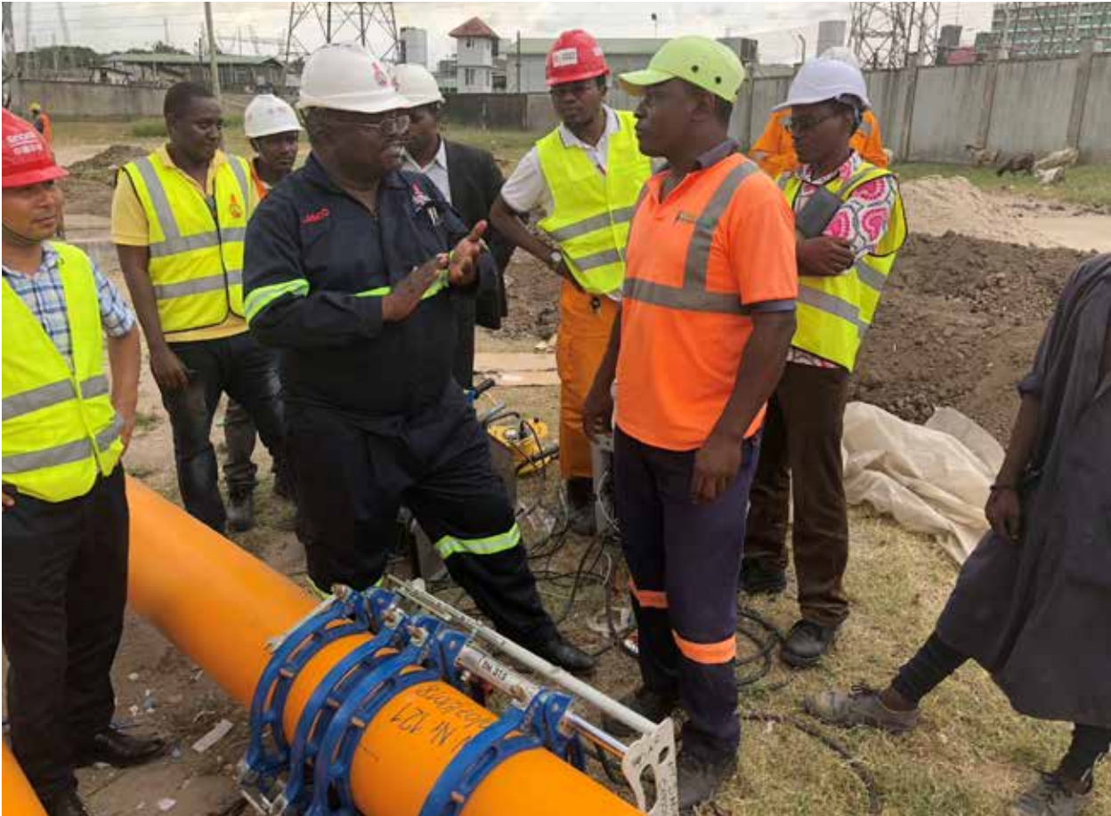
Figure 17: Natural gas distribution project implementation
